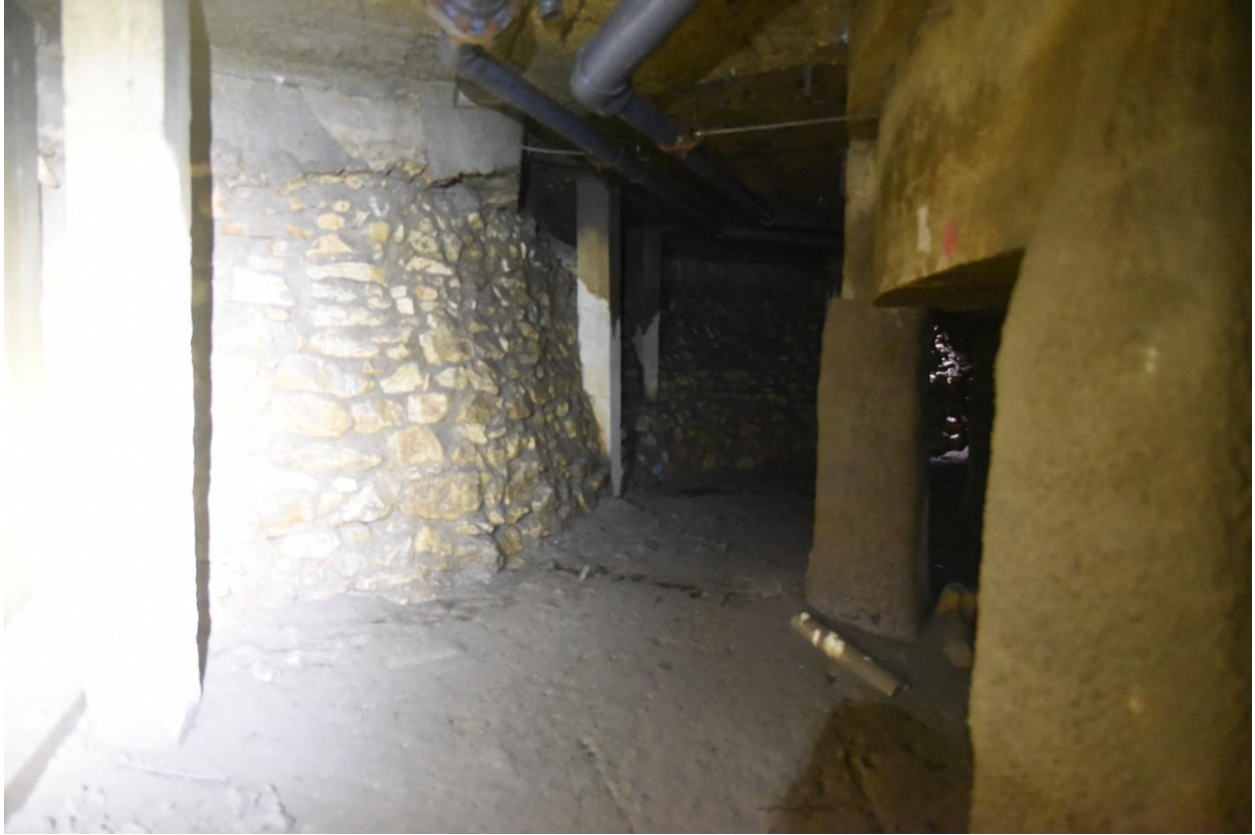
Figure 5. Under the pool deck, looking south toward the south corner. Concrete retaining wall on the left; stone masonry retaining wall ahead, center; pool structure on the right.
