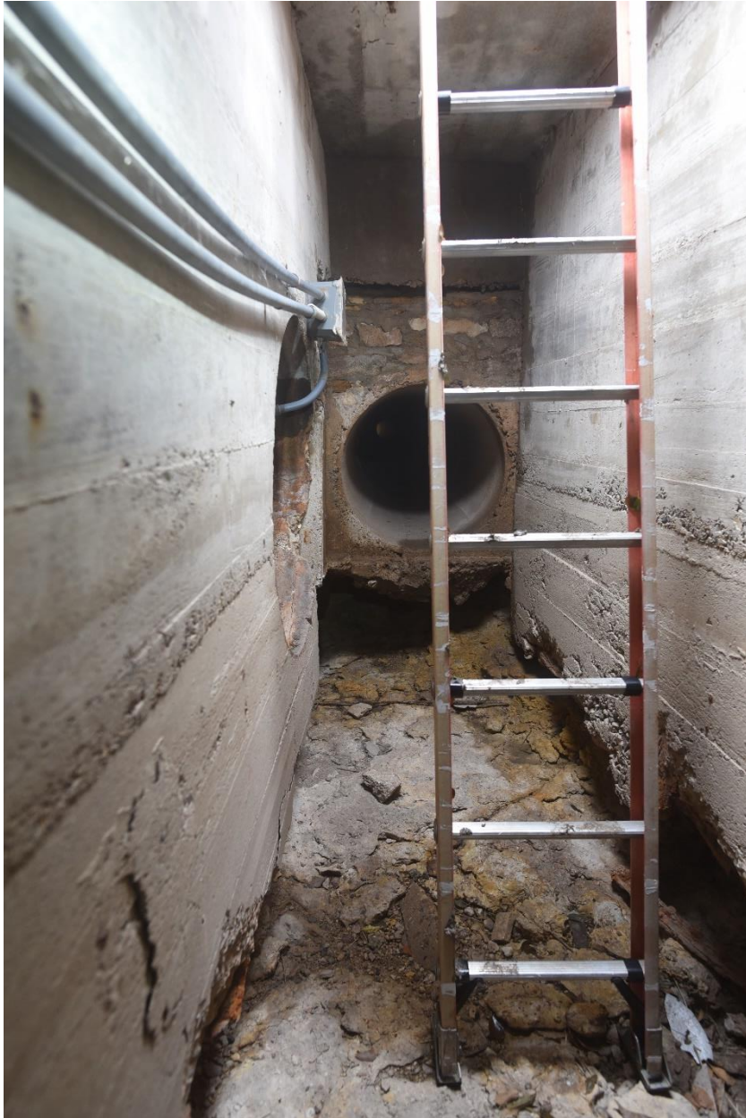
Figure 10. Inside the box culvert on the west side, looking south. The pipe ahead connects to the main spring (Big Chief spring). The opening to the pool basin is on the left. A fissure in the rock is near the bottom of the ladder. Below the pipe ahead, soil is washed out below the pipe and to the left of this is an area of collapsed stone masonry wall (not visible).
