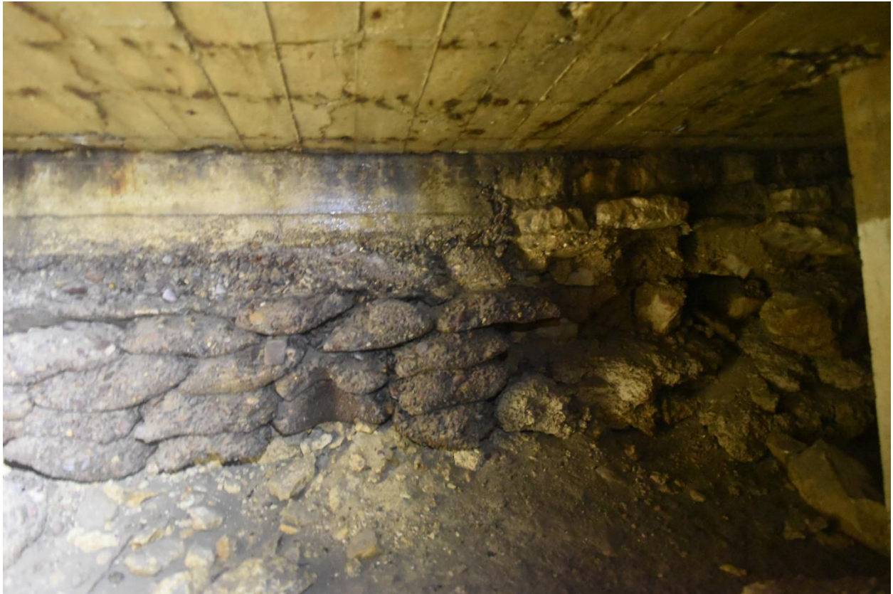
Figure 13. Wall repair using bagged materials.
