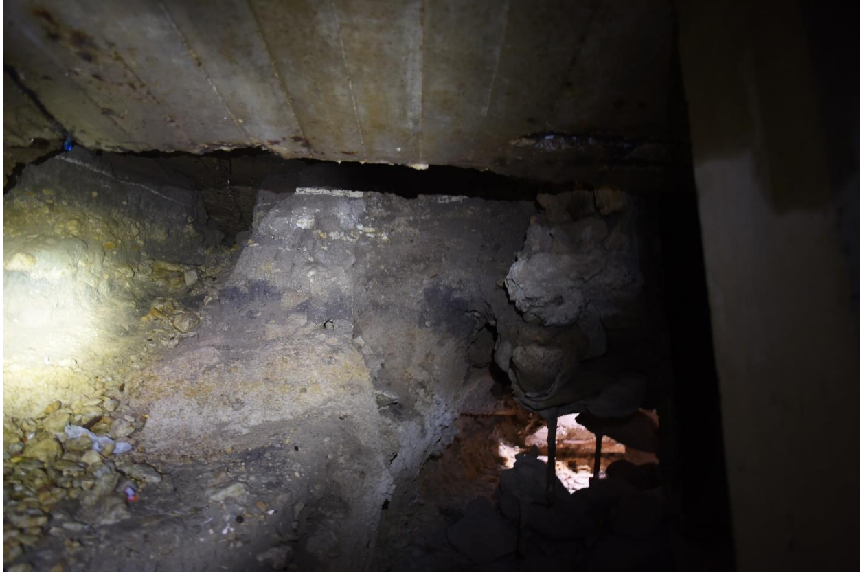
Figure 14. Retained area on west side of basin. The location of the collapsed wall is on the left. The open fissure into the concrete box is on the lower right.
