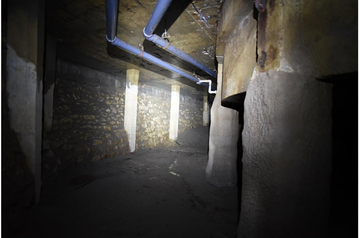
Figure 6. Looking west from the south corner. Stone masonry retaining wall on the left and ahead; pool structure on the right.
